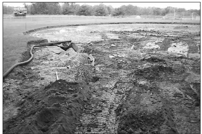
New Field Drainage Pipes at Major League
